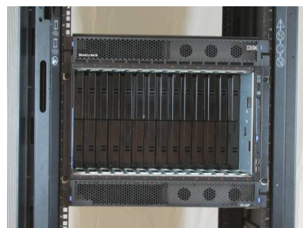
Figure 7C: The IBM chassis installed on the rails.
